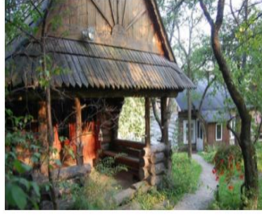
Natural building in Bhrugu Aranya, Poland
